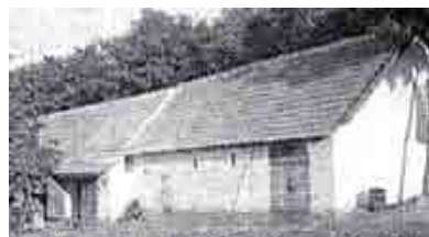
George Zimmermann's home place in Kaschpalat, 1938. The barn was made of adobe; the other buildings and the cellar were of shell-stones, found only in the Black Sea area; the roof tiles were made of cement. Oskar Zimmermann grew up here.
