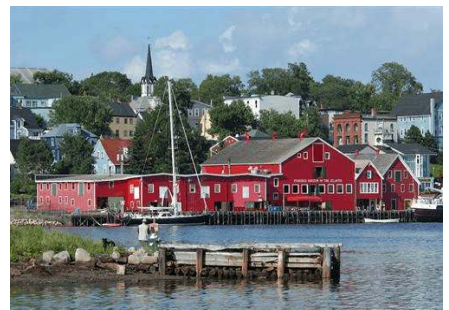
The Fisheries Museum of the Atlantic in Lunenburg is currently undergoing an engineering assessment, part of an ongoing process designed to ensure the long-term preservation of the facility's buildings.
