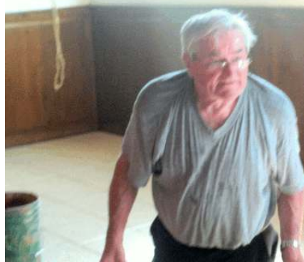
Werner Bachhuber grouting
